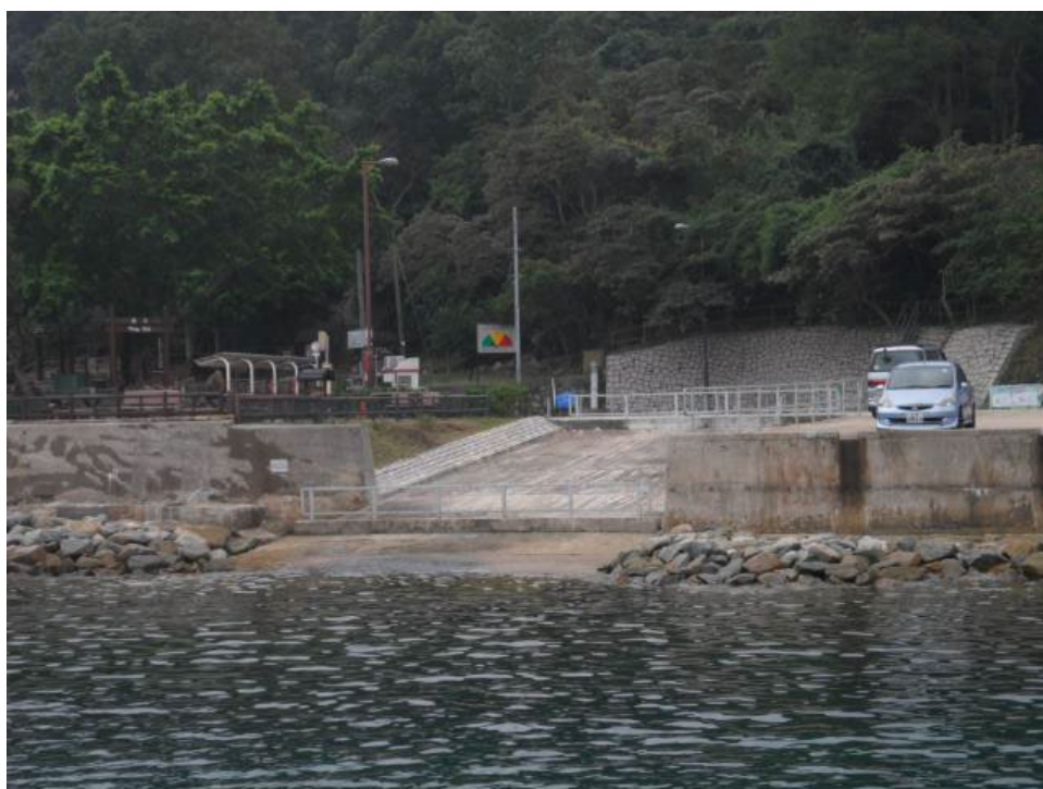
Example: Wong Shek Slipway
