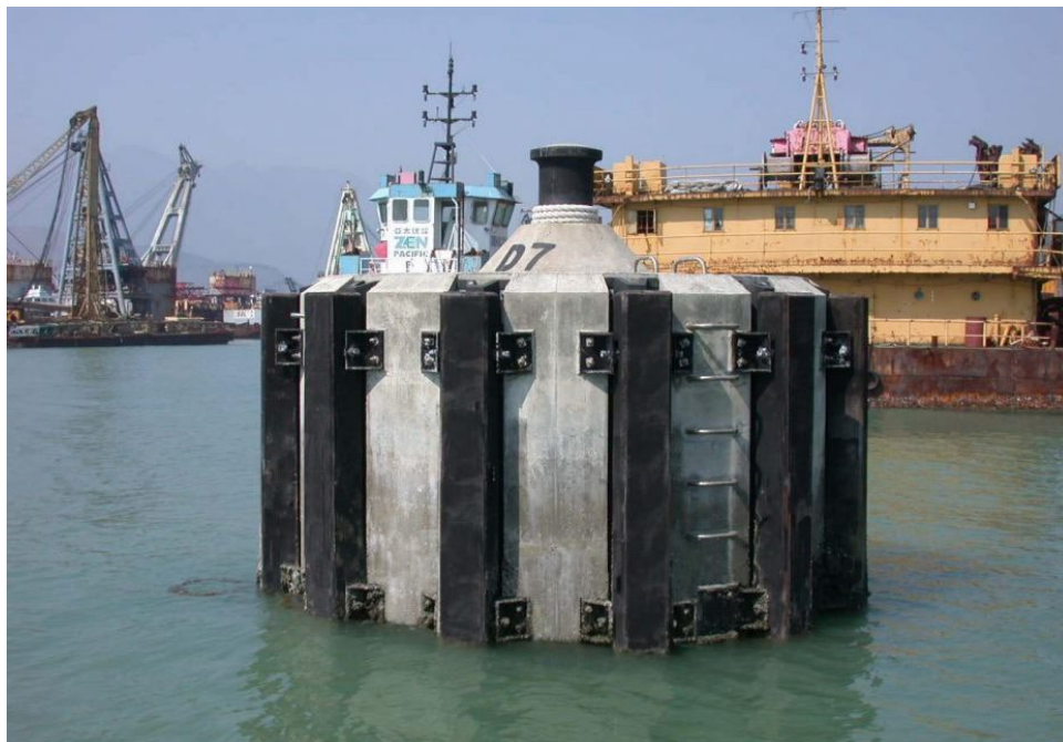
Example: Mooring Dolphin in Hei Ling Chau Typhoon Shelter
