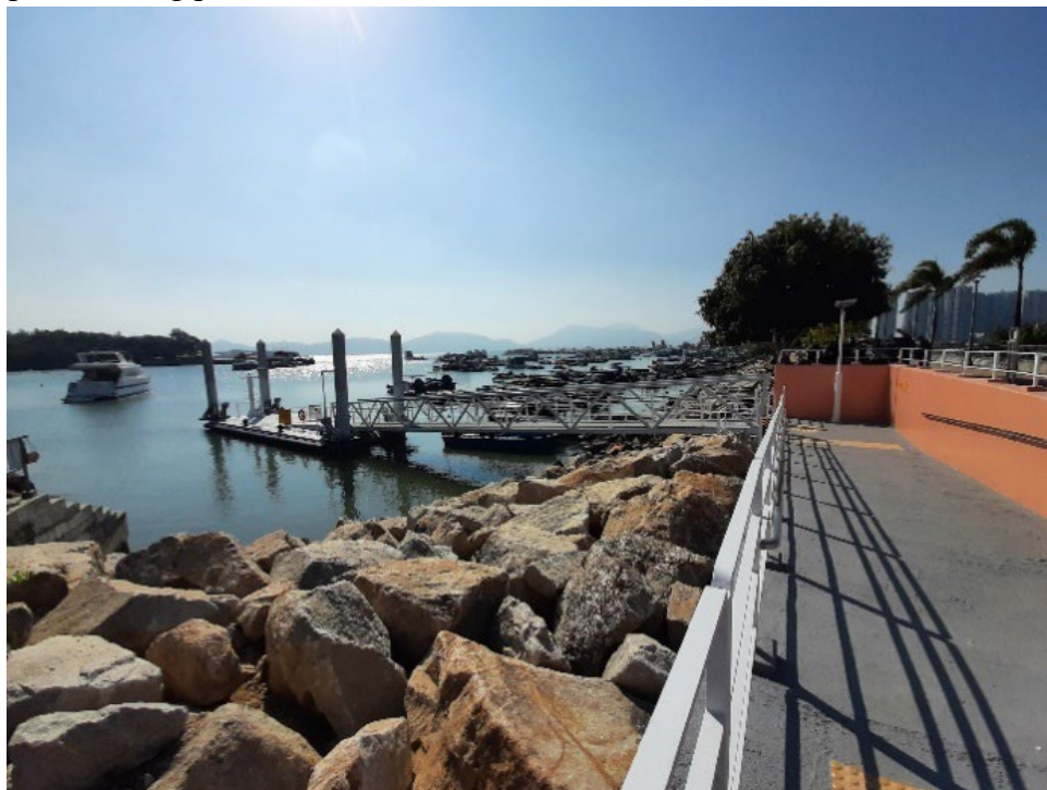
Example: Floating pontoon at Tuen Mun Area 27
